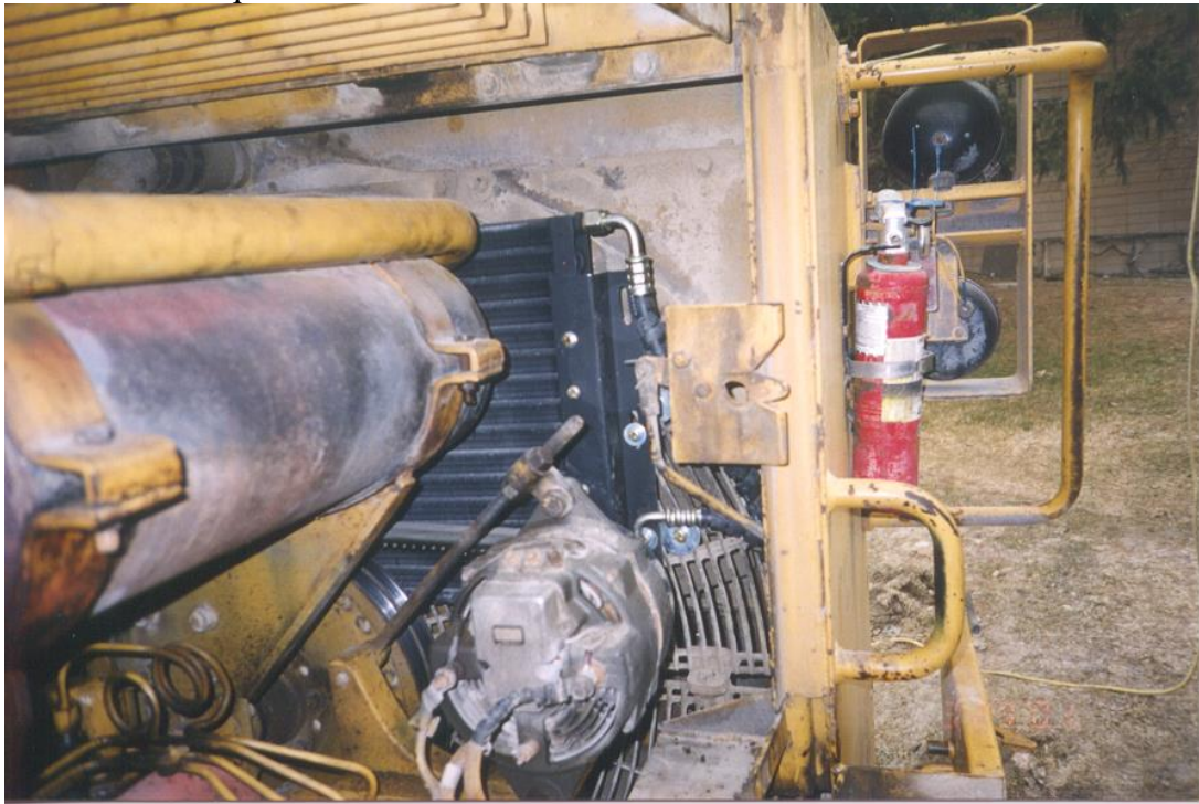
Condenser as viewed from left side.
