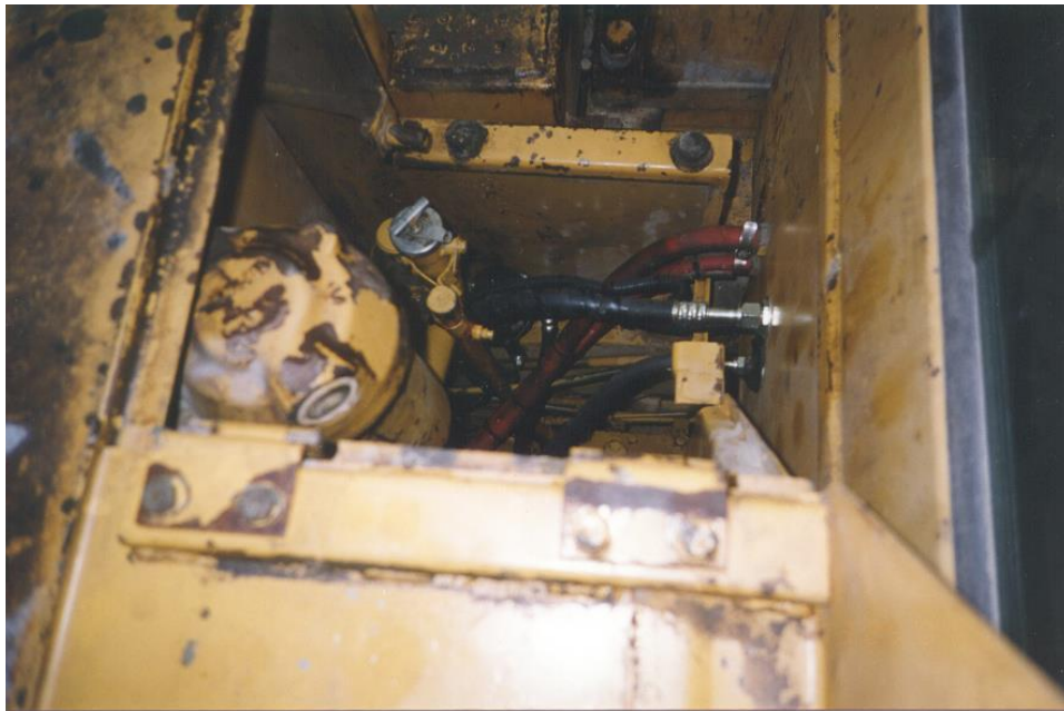
Drier in place with hoses.
